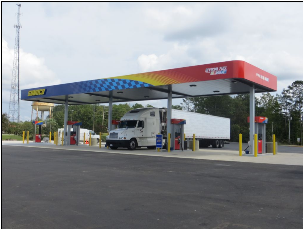
New diesel pumps
