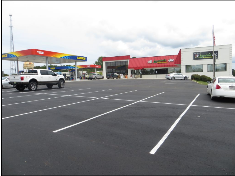
New completely resurfaced and expanded parking lot
