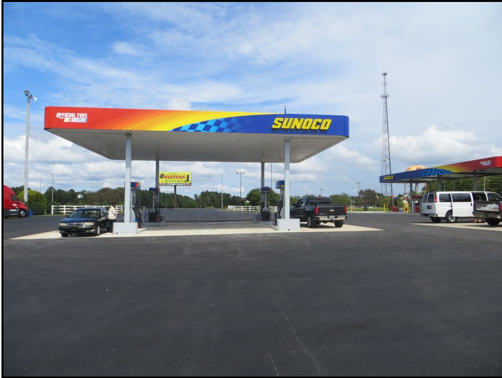
New gasoline pumps
